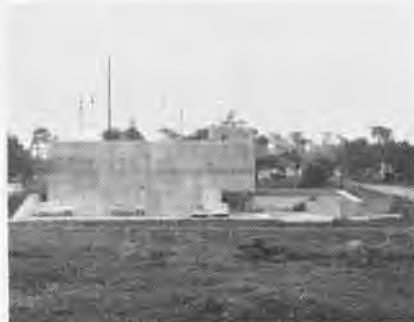
THIS NEW concrete structure houses one of the finest land-based CIC's. It is the Naval Air Intercept Training Facility, Point Pinos, Calif., near Monterey which gives special training to squadrons in the San Francisco area.
