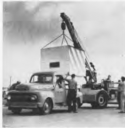
A PIGGY BACK TRAILER brings "a home away from home" for the men who guard aircraft wreckage day and night until investigations are complete. Designed by NAAS Chase Field, Beeville, Texas, and made by "C" Maintenance unit under the direction of LCdr. Edwin van Biesbroeck, the piggy back provides guards with an "on-the-scene" coffee lounge and sleeping quarters. It was made of scrap pipe and aluminum sheeting. Besides the quick mounting, the trailer but features open-side screen ventilation, two bunks, and a mounted two-gallon thermos jug.
