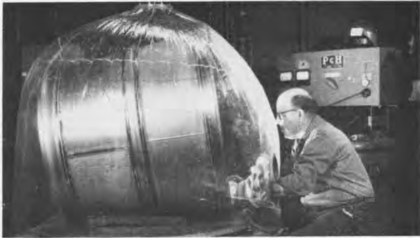
TO AVOID contamination by oxygen and nitrogen during the welding process, alloy titanium is joined in a plastic bag filled with argon gas, a new technique to increase use of titanium.
