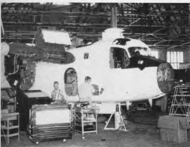
WORKMEN INSTALL AND CHECK ONE OF THE ELECTRICAL SYSTEMS
