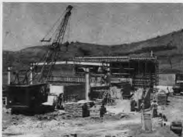
CONSTRUCTION MEN ERECT A NEW BUILDING FOR MISSILE BASE
