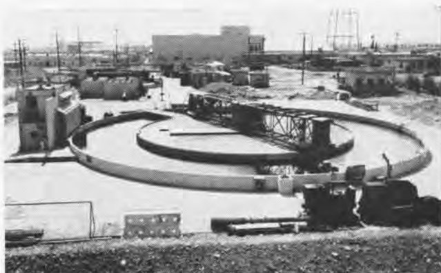
AEROJET USES THIS RING CHANNEL UNDERWATER TEST FACILITY
