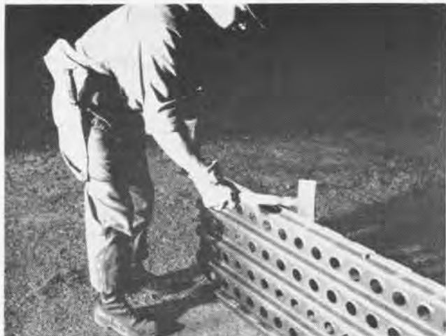
7TH MARINES ENGINEER BENDS HOOKS ON MATS FOR PROPER FIT
