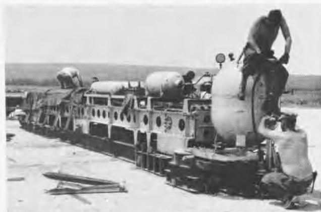
TWENTY-TWO STAKES ARE DRIVEN IN TO ANCHOR MOREST IN PLACE
