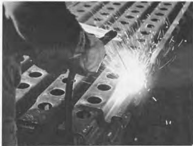
THE LAST PIECE OF MATTING IS CUT TO SIZE FOR LANDING FIELD
