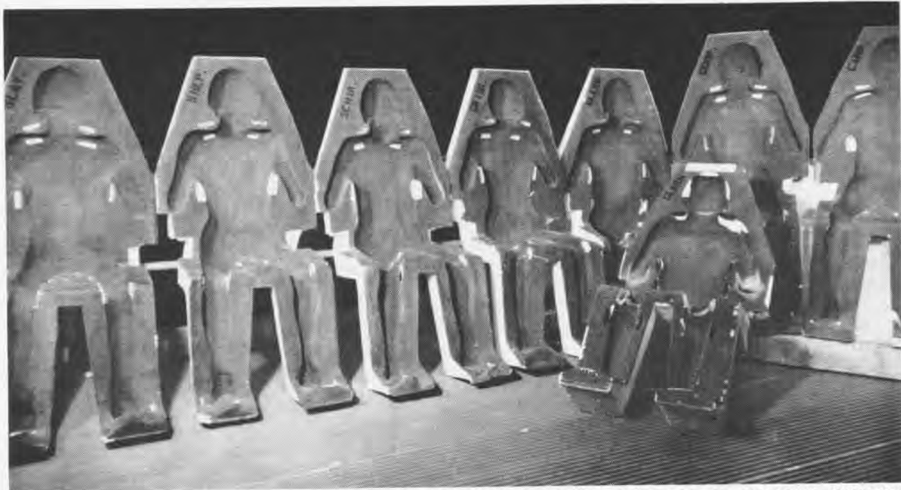
SPACE COUCH QUORUM AT NAVY'S AMAL SUGGESTS EGYPTIAN SCENE. EACH WAS MOLDED TO FIT INDIVIDUAL ASTRONAUT
