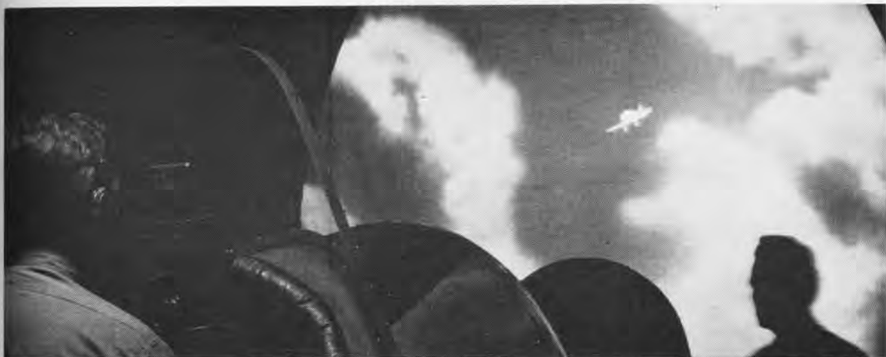
TRADEMARK OF SIMULATION effort in WW II was gunnery trainer. Ability of pilots to use airplane as gun platform was fundamental consideration given earliest attention by de Florez team. With realistic training on ground, Navy pilots downed enemy at rate of 22-1.
