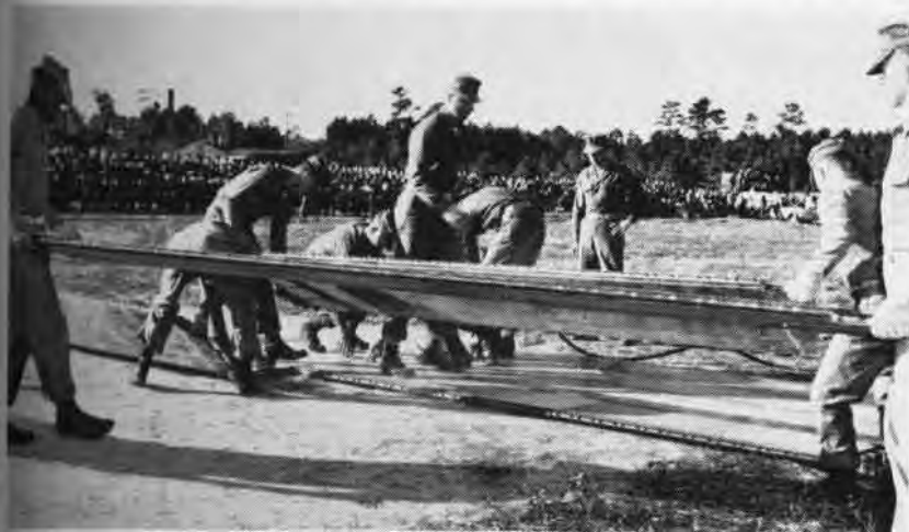
IN 15 MINUTES, COMBAT ENGINEERS LAY DOWN 50-FOOT ALUMINUM RUNWAY SECTION
