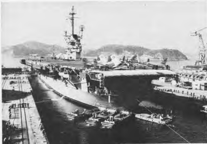
UNUSUAL STERN FIRST entry into Yokosuka dry dock is made by USS Hancock. Only one other carrier in the history of the Ship Repair Facility there had made a stern first entry before Hancock. That was USS Bennington in 1936. Hancock was docked in her unusual position to permit work on after part of the ship. Stern section of angle deck carriers is more easily available to workers and to crane service in that particular position. Note LCVP's in tug roles.
