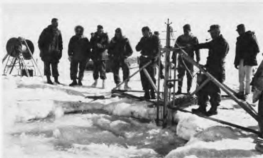
MOTION CREATED BY AQUA THERM UNIT CAUSES WATER TO GNAW AWAY AT THICK ICE
