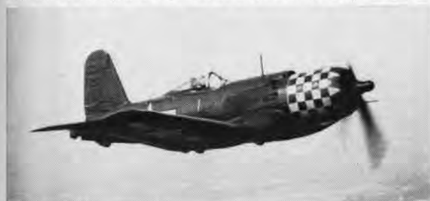
GOODYEAR F2G's were Corsairs redesigned with 3000-hp P&W Wasp Major engine, weighed 13,000 pounds, reached 431 miles per hour.
