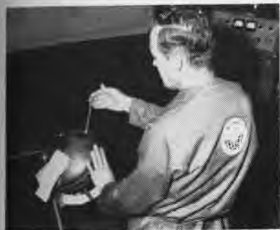
TUBE IS ATTACHED TO LOX CONTAINER
