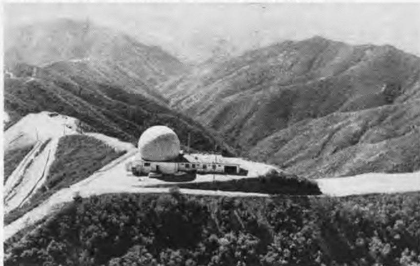
EL TORO'S NEW SKY-SCANNER radar, the eyes of recently activated Radar Air Traffic Control Center (RATCC), sweeps the Southern California skies. It is located atop 4008' Pleasant's Peak, 12 miles northeast of the air station. Radar information from the mountain top is "piped" to the Center on the air station, which is jointly manned by FAA and Marine Corps personnel. The radar antenna, revolving six times a minute, has a surveillance radius of 200 miles.
