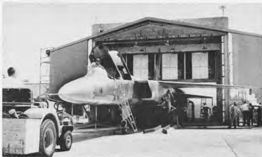
NEW SOUND ABATEMENT building at North American, built at cost of $1/4-million to reduce sound level of jet engine run-ups by more than 90 percent, has been put into use. It is built of reinforced concrete with walls from 12 to 18 inches thick and will be used to permit flight line crews to perform their work with the A3J more effectively. The 76x336-foot structure will house the rear section of the A3J's fuselage in which two GE-J79 turbojets are mounted.
