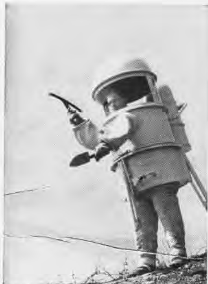
WORKING MODEL of a two-piece lunar exploration suit is tried out on a moon-like hill on Long Island. Developed by Republic Aviation, the suit is meant to be the astronaut's working clothes once he reaches the moon.
