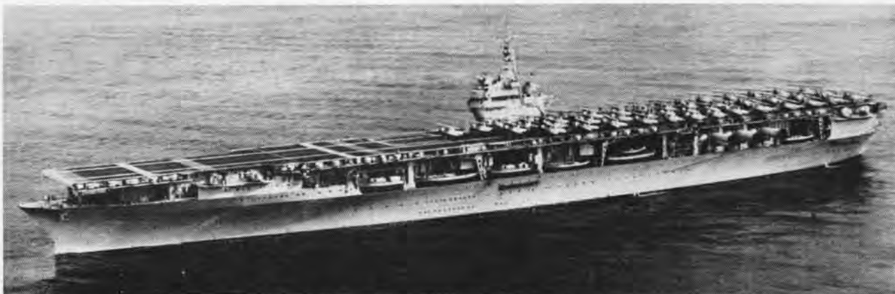
THE 14,500-TON RANGER was the first ship to be built as an aircraft carrier from the keel up in contrast to its predecessors which were
