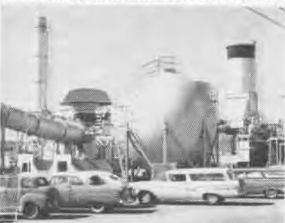
FT MUGU'S "Big Blow," a wind tunnel capable of speeds six times the speed of sound, is powered by power plant of USS Independence (C-122). Atom-bombed at Bikini, she "steams on," her large funnel in use at right.
