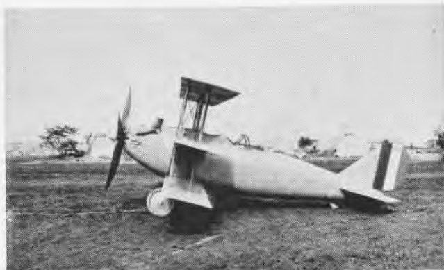
CURTISS 18-T "Kirkham Fighter," 350-horsepower Curtiss-Kirkham engine, was 2920-lb., two-seat triplane credited with 162 mph in 1919.
