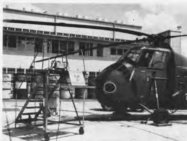
ROTOR BLADE spars on HSS/HUS helicopters were x-rayed after the spar defect was found in one of the type. Film is placed atop rotor blade.
