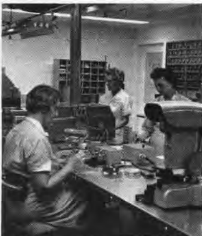
IN INSTRUMENT bearing shop, everything is small-scale to accommodate miniature bearings.
