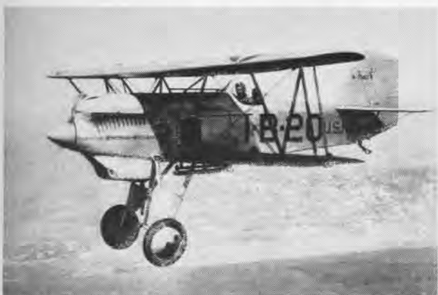
ONE OF THE FAMOUS Curtiss Hawks, the F6C-3, entered service in 1926, weighed 2960 lbs, reached 165 mph with 425-hp Curtiss D-12.
