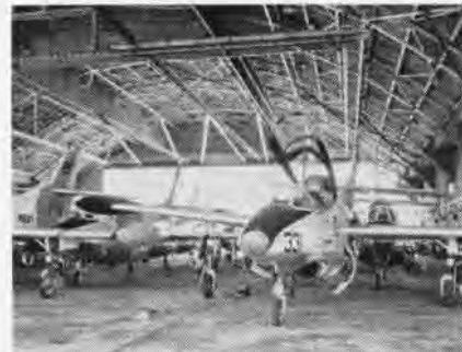
HIGH-LOW OLEOS permit packing "Buckeyes" solidly in Forrest Sherman Field hangar during Hurricane Donna. Chief Mayo, Training Squadron Four's Aircraft Maintenance Chief is credited with the "cockeyed" suggestion.
