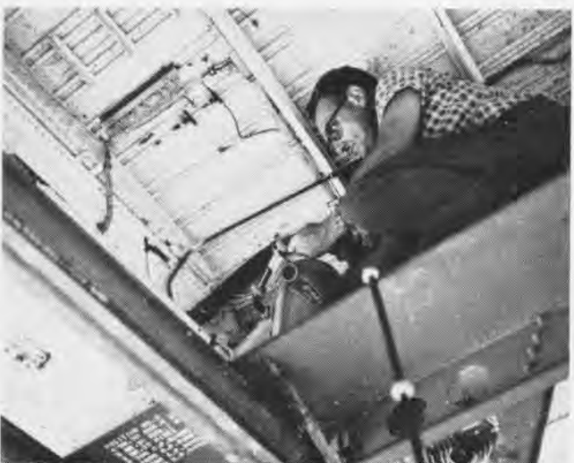
X-RAY HEAD is positioned for a view of F4D leading edge slot track. With radiography, defects can be spotted without taking plane apart.
