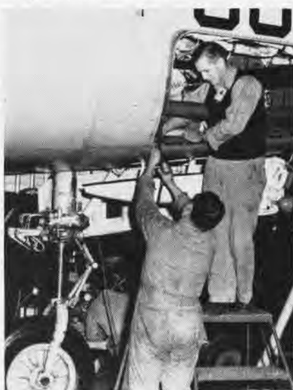
FINAL TOUCHES ARE PUT ON NOSE SECTION
