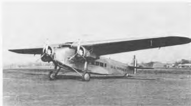
ORIGINALLY DESIGNATED TA's, Atlantic (Fokker) tri-motor RA's served with Marines. RA-4 had P&W Wasps; nose was later lengthened.
