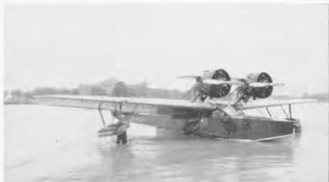
DOUGLAS DOLPHIN amphibians were Navy and Marine Corps RD's. Landing gear on RD-3 was raised to clear water, not to reduce drag.
