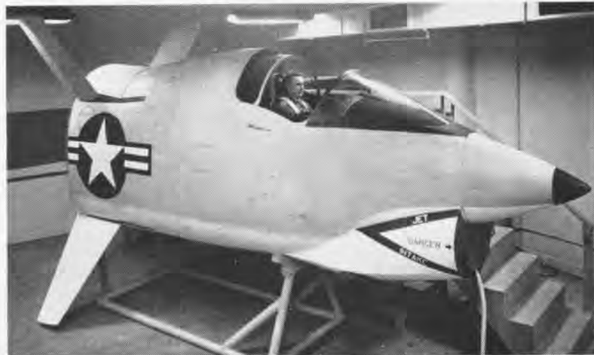
MOCK-UP OF 'OSCAR' (OPTIMUM SURVIVAL CONTAINMENT AND RECOVERY) CAPSULE
