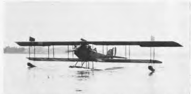
STANDARD SEAPLANE trainer, WW I, and for many years after, was Curtiss N-9, built with different engines and by different companies.
