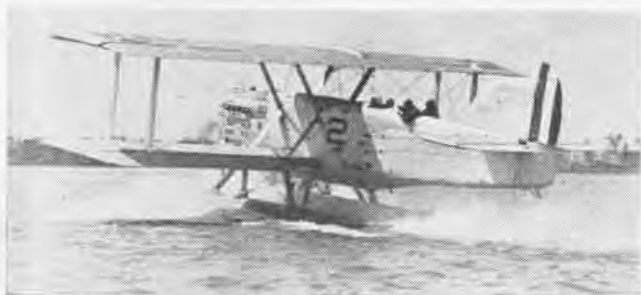
LONG RANGE SCOUTS were the SDW's of 1924, modified from Douglas DT's by Wright, incorporating the Wright 625-horsepower T-3 engine.
