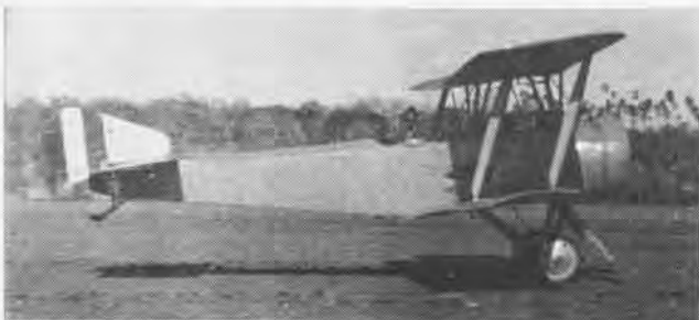
TAKING OFF at Guantanamo is a WW I British Sopwith 1½ Strutter, converted to a Navy shipboard type with hydrovane and flotation gear.
