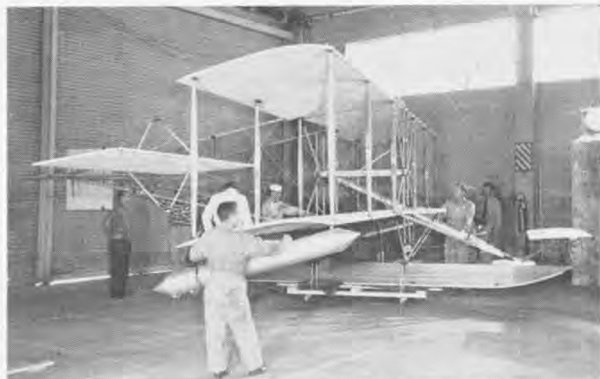
A-1 FRAME, FREE OF JIGS, IS SPOTTED FOR ENGINE INSTALLATION AT MARINE CORPS DEPOT
