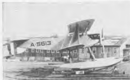
1922 AEROMARINE , an experimental seaplane scout, was powered by 300-hp Wright Hisso.
