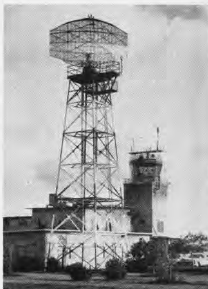
MIRAMAR FACILITIES , here the radar antenna and control tower, serve fighter squadrons.
