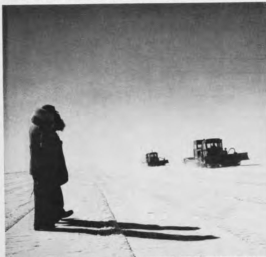
JAY R. BERRYMAN, PH1, SHOOTS OPERATIONAL PICTURE OF ICE RUNWAY CONSTRUCTION
