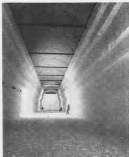
TAYLOR PICTURES BYRD STATION TUNNEL
