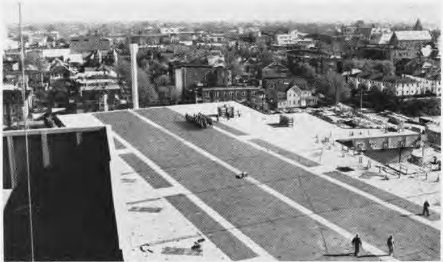
AT FIRST GLANCE , this looks like a photograph of a "street that leads to nowhere." A second glance however, proves it to be the aft end of the flight deck of the carrier Enterprise (CVAN-65), towering over the waterfront of Newport News, Va. Squad of Marines adds to the illusion.
