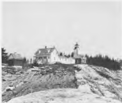
PEMAQUID Point lighthouse, overlooking Gulf of Maine, houses monitoring equipment.
