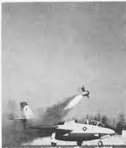
THESE GROUND-LEVEL TESTS OF THE ROCKET SEAT IN THE T2J BUCKEYEWERE PART OF NORTH AMERICAN AVIATION'S TEST PROGRAM
