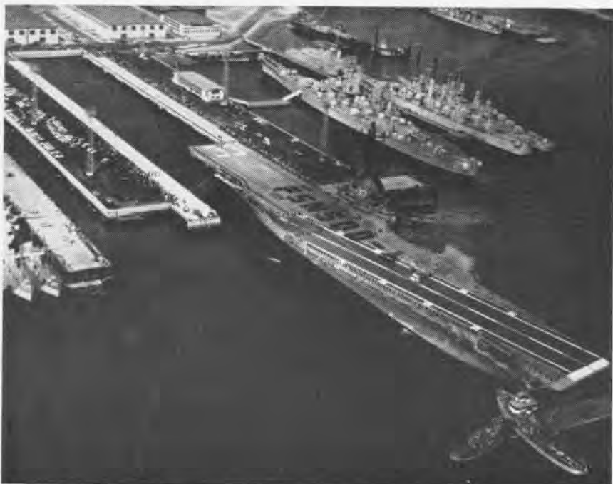
ALMOST DWARFED , USS Kearsarge (CVS-33) slowly steams into the world's largest drydock at Puget Sound Naval Shipyard, Bremerton, Wash. The 14-acre dock (DD-6) is 1180 feet long, 180 feet wide, 61 feet deep, and has a water capacity of 88,000,000 gallons. The "Mighty K," which had the honor of participating in the dedication ceremonies, recently completed a six-month conversion at the yard. Capt. L.E. DeCamp is C.O., and home port is Long Beach.
