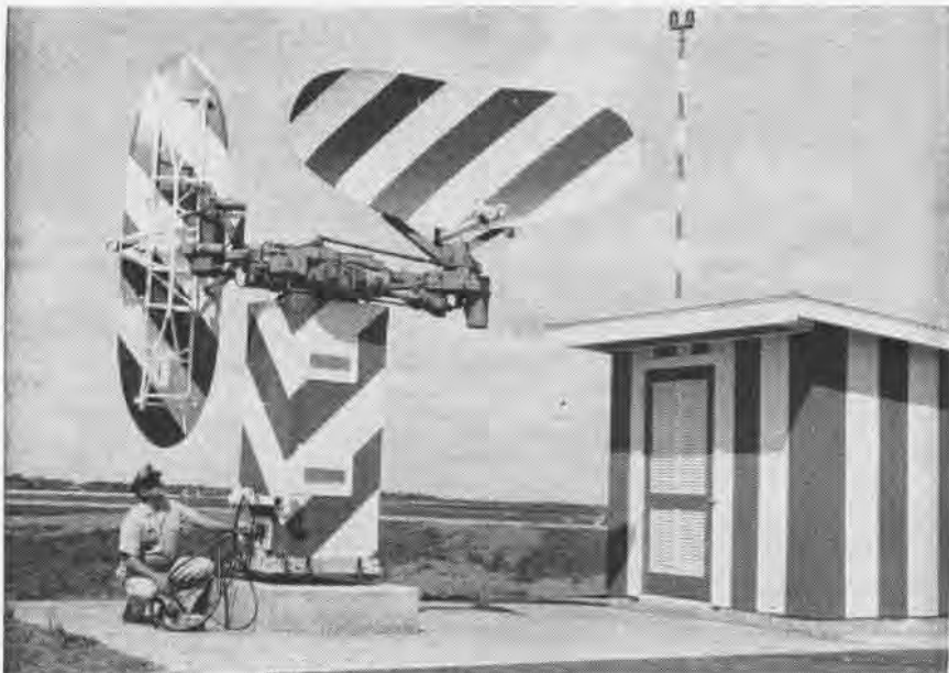
G. R. WHITE, ATC, makes a final inspection of FPN-36 "quad" radar system now in service at NAS Cecil Field, Fla. The new radar system will allow GCA approaches on all four of Cecil Field's runways from a single control point. It permits instantaneous shift of runway control. The mobile trainer unit, which was formerly in use, could control only one pair of runways at a time, and shifting the unit to the other pair took as much as 30 minutes.
