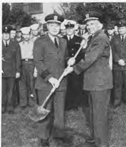
CAPT. W. P. TANNER, Jr. , Los Alamitos C.O., is handed shovel by Cdr. J. W. Hurnblad, C.O. of Naval Air Reserve Electronic Training Unit, to break ground for extension to the building that the unit is housed in.
