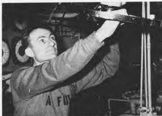
IN PUMP ROOM, LOUIS PASTELL, ABF2, STARTS AVGAS TO TOPSIDE
