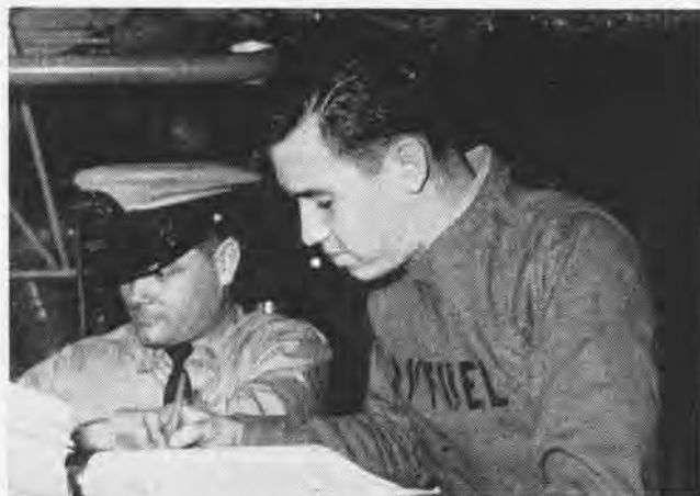
PAPERWORK IS DONE BY EDWIN CULVER, ABFC, AND JOHN HICKMAN
