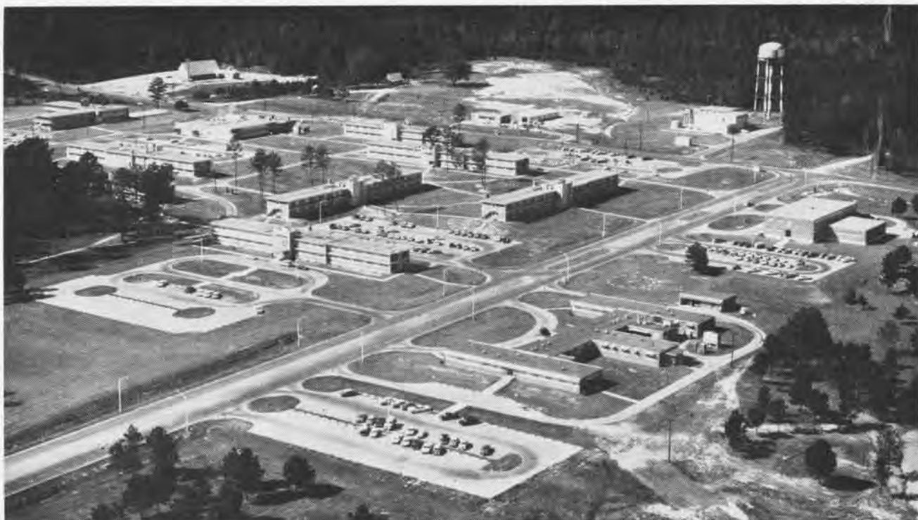
THIS COMPLEX of buildings in the administrative section at Meridian is located three miles away from the noisy flight operations area. All of these structures are of a permanent nature, modern in design. Formally commissioned in July 1961, base is a CNABATRA unit.
