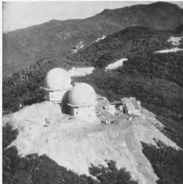
TWIN RADAR TOWERS on a mountain top near the station provide information for safety control of the missile-firing air spaces in the area.
