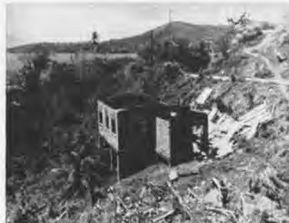
THIS HILLSIDE dwelling, photographed by a U.S. Navy plane on mission, was badly hit.
