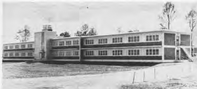
THE ENLISTED MEN'S barracks provide comfortable living quarters for Meridian sailors. Spaces are designed for four people per room.
