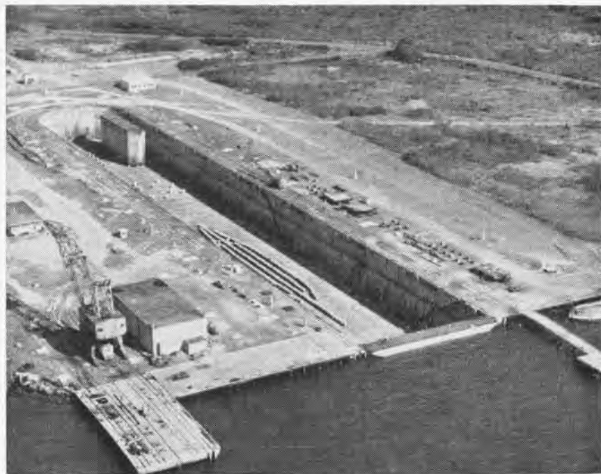
ONE OF THE WORLD'S LARGEST , the dry dock at Roosevelt Roads, 1088 feet long, can accommodate any ship in the world. It was built during WW II and serviced ships through the war.
