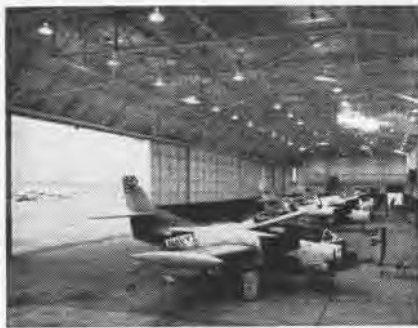
DOUBLE-CANTILEVER type hangar provides excellent maintenance facilities for Buckeyes.
