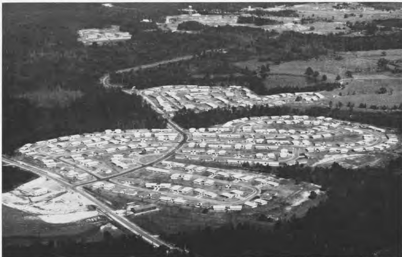
THE CAPEHART HOUSING section is situated two miles west of the administration area and five miles from the runways. The units are made of brick and have from two to four bedrooms. More than 230 of the units are assigned enlisted men; 88 are set aside for officers.
