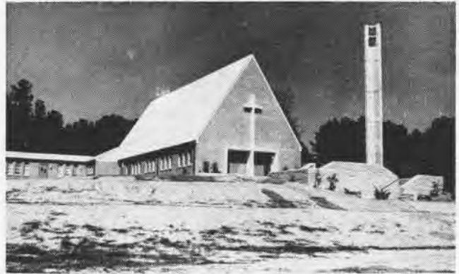
MODERN CHAPEL which was recently completed is located a short distance from administration area. First services were held this autumn.
