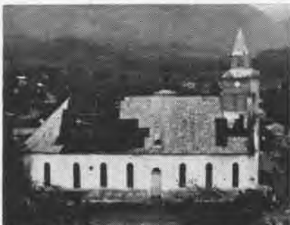
ALTHOUGH ROOF was partially torn off, steeple of church withstood Flora's wild onslaught.
