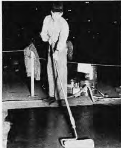
SAILOR SMOOTHS SURFACE WITH ROLLER
