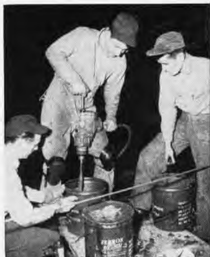
FERROX ABRASIVE MIXED WITH NON-SKID
