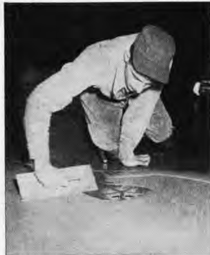
TROWEL AIDS IN SPREADING THE MIXTURE
