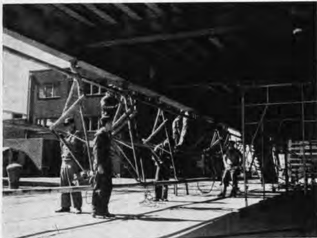
VIEW FROM the bottom of USS Independence shows men installing new aircraft elevator safety nets during overhaul at Norfolk Navy Yard.
