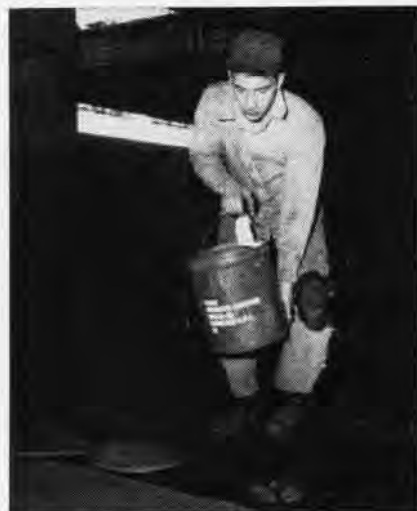
NON-SKID IS Poured ONTO HANGAR DECK
