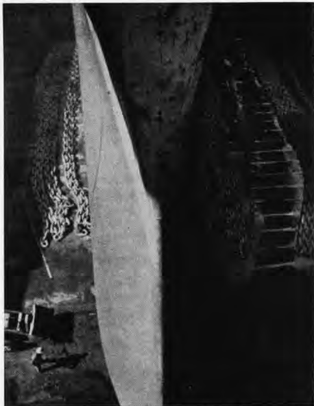
ANCHOR CHAINS line the exposed hull in Norfolk Navy Ship Yard. Each link in the chain weighs 360 pounds, helps hold 30-ton anchors.
