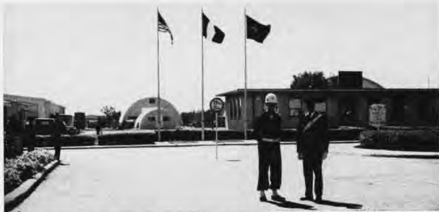
FACILITY AT SIGONELLA, SICILY, IS MAINTAINED WITH PERMISSION OF ITALIAN GOVERNMENT
