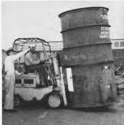
HANDLING procedures in moving a "canned" engine are checked by D. M. Hood, ABFC.
