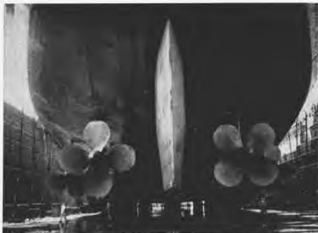
WORKERS ARE DWARFED by the huge cloverleaf props and rudder of Champ as arrangements are made to start sandblasting her bottom.
