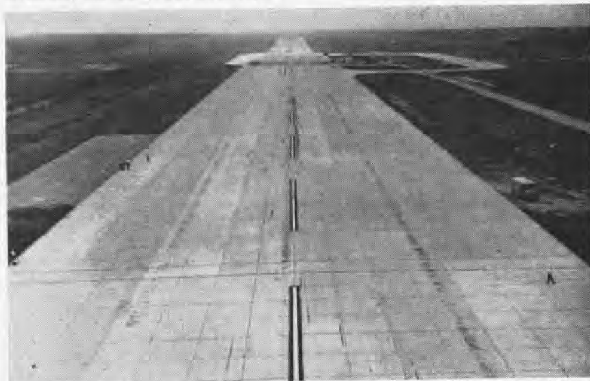
LONGEST RUNWAY in New Jersey is Lakehurst's recently extended, 12,000-ft. strip used by the Naval Air Test Facility (Ship Installations). Completed last May, the runway will better serve heavier and faster jet aircraft in test activities. At right is diversion strip which has carrier landing deck dimensions and permits rapid turn-around time for planes evaluating new equipment. Newest steam catapult and an angled-deck strip are also located in test area.
