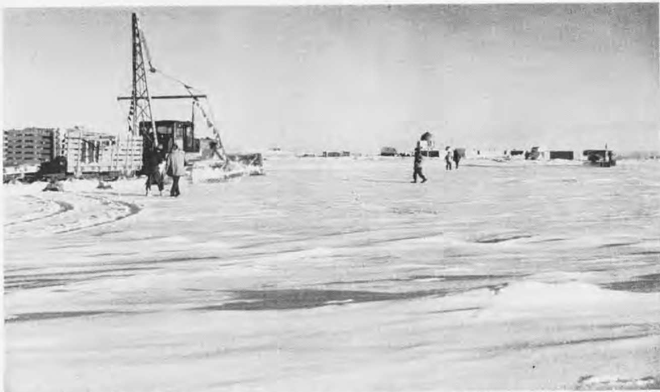
EIGHTS STATION on a plain at the foot of the Palmer Peninsula is reached by a traverse party after an 888-mile trek from Byrd Station. A D-8 tractor was hauled to prepare snow surface for modules. All other equipment, personnel, stores were airlifted or airdropped.
