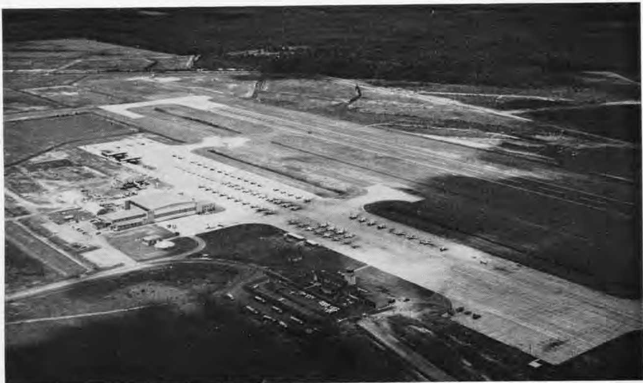
THE NAVAL AIR STATION at Glynco, Brunswick, Ga., had its beginnings as a Naval facility in World War II when airships used it as a base from which they flew thousands of hours of patrols searching for German U-boats. Not a single Glynco airship was lost while on duty.
