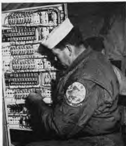
ELECTRICAL components of gear aboard are checked in flight by J. G. Strickland, AT1.
