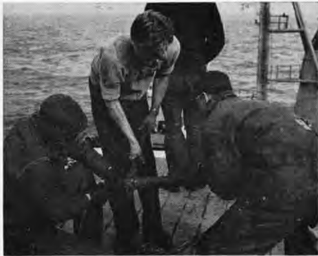
REPAIR WORK on a hose is accomplished by Dixon, Edward J. Pollick, AN, and Richard L. Ponzini, AN, on flight deck of "Champ."
