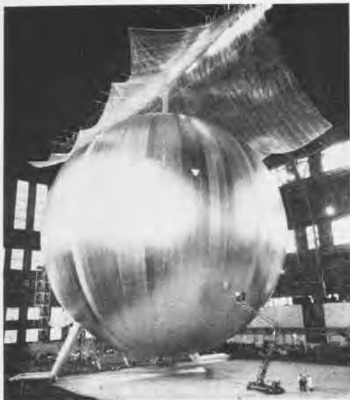
AT HANGAR ONE, NASA carried out various types of tests on the 135-foot-diameter Echo II satellite.
