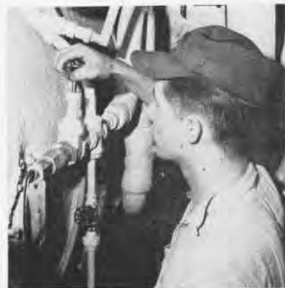
W. H. BROWN, MM3, increases pressure in one of the main salinity cells in CVA-34 .
