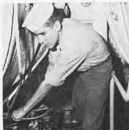
D. TRUJILLO, FN, opens valve to advance salt water to the next stage of evaporation.
