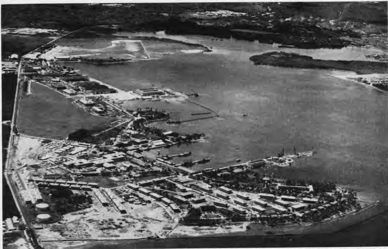
IN 1941, COCO SOLO, STRATEGICALLY LOCATED NEAR PANAMA CANAL, WAS BUILT UP SPEEDILY BY SEABEES AS AIR STATION AND SUB BASE
