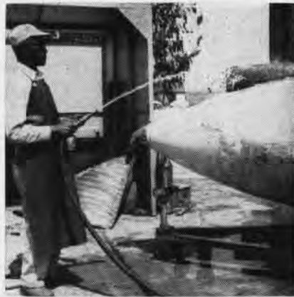
BEFORE THE WORK gets underway, Rudolph Jones washes down the damaged radome cone.
