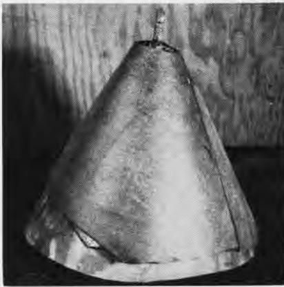
THIS MOLD was installed in the nose cone before repair to insure proper contour.
