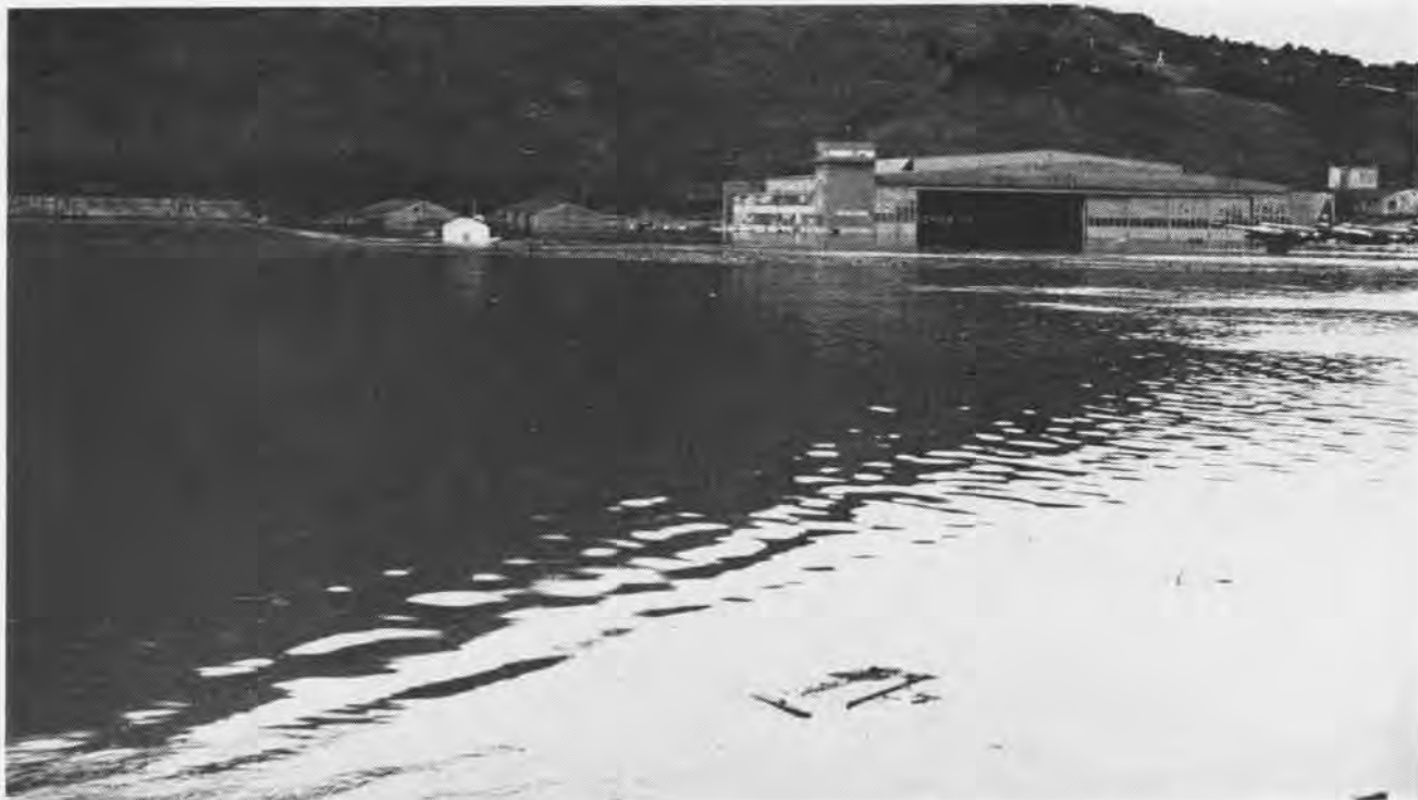
THREE TIDAL WAVES , one immediately after the earthquake, deluged the Kodiak station ramp which leads into Old Woman's Bay. The first crested at 22 feet above the area's low tide mark; the second (at 2200) crested at 25 feet; the third wave, early the 28th, at 30 feet.
