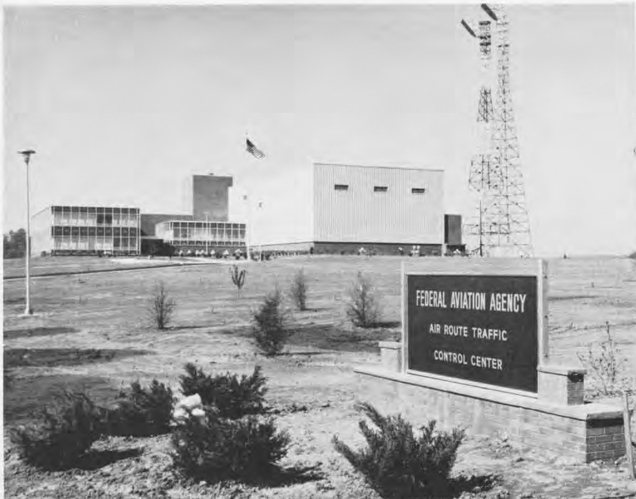
WASHINGTON ARTCC is located in this modern structure at Leesburg, Va. Hub of operations is the main control room (C). Administrative offices are on left and radar microwave towers stand at right. Dedicated last June, the Center has 500 specially-trained employees.
