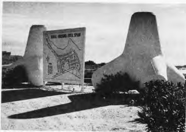
AS FAMILIAR to NS Rota as the Empire State Building is to New York are these giant tetrapods, specially designed to control tidal flow.
