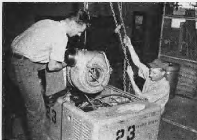
'BRAVES' N. W. Ream and J. M. Thomson, both AA's, work together in pulling a GTC 85-72 compressor unit during periodic inspection.
