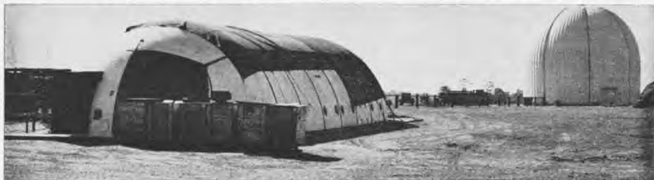
OPERATIONS SHELTER is equipped with the eyes of the new AN/TPS-34 tactical radar system while 150 feet away, the 47-foot radome conceals the cars. The radome, exposed to winds of 75 knots and gusts up to 90 knots, withstood them perfectly with no ill effects.
