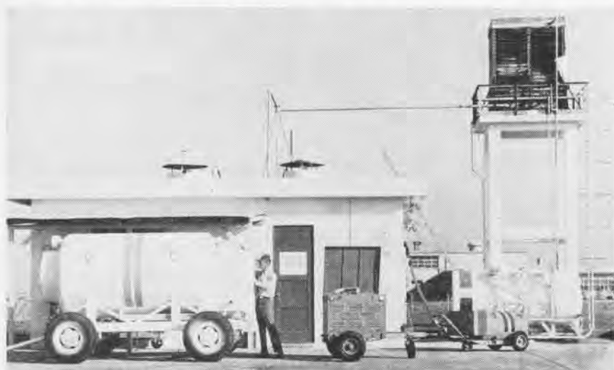
SIGONELLA'S LOX PLANT is manned 24 hours a day as men monitor production phase of LOX called "on steam." Here, man checks one of 500-gallon portable tanks used to carry LOX.
