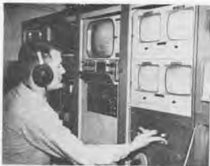
CONTROLS of the PLAT system are operated in the Forrestal by man in OC Division.
