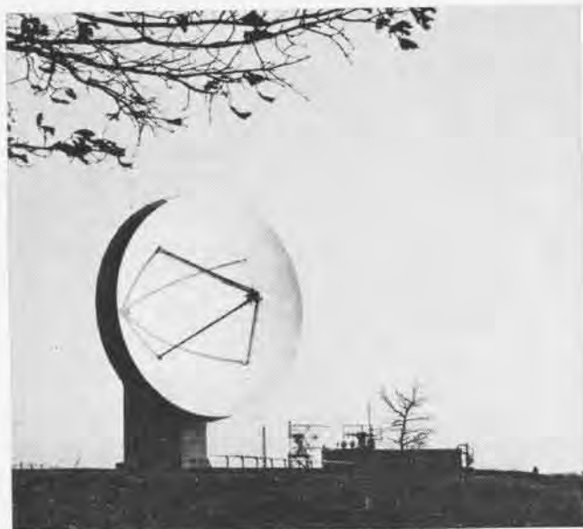
THE FIRST ANTENNA for Navy's navigational satellite system was installed at Johns Hopkins' Applied Physics Laboratory near Baltimore.
