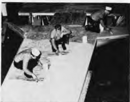
NON-SLIP PAINT IS APPLIED TO THE DECK
