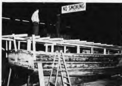
STERN VIEW SHOWS FLIGHT DECK BRACES
