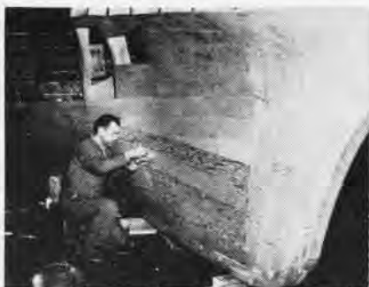
BOW EXTENSION ADDED SIX FEET TO HULL
