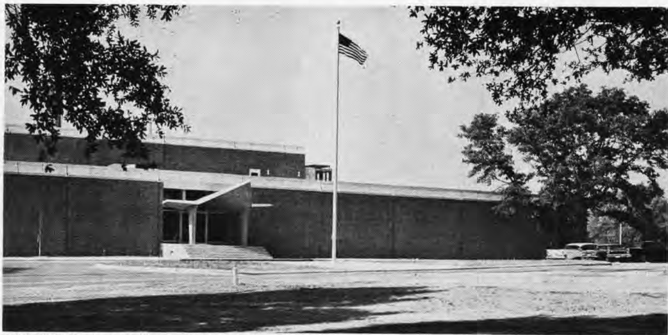
FRONT VIEW OF the $3.5 million two-building complex at the U. S. Naval School of Aviation Medicine at NAS Pensacola, Florida. The newly constructed facilities consist of two windowless, air conditioned buildings with a total combined area of 90,000 square feet.
