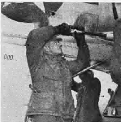
BLAST DEFLECTOR on Skyhawk 's 20mm guns is adjusted by Ordnanceman Daugherty.
