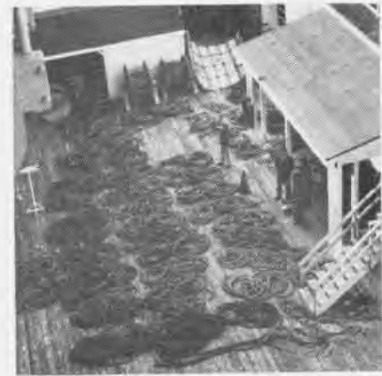
SOME OF EIGHT miles of 1½-inch deperming cable is laid out at Craney Island facility.
