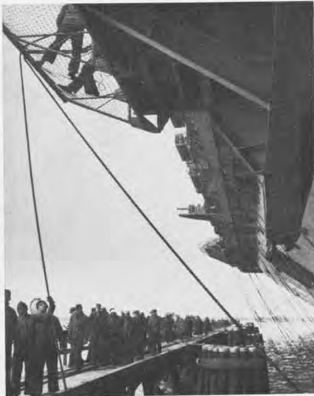
AMERICA CREW MEMBERS rig deperming cables around carrier's girth. With a cable required for every 15 feet, working parties were busy.
