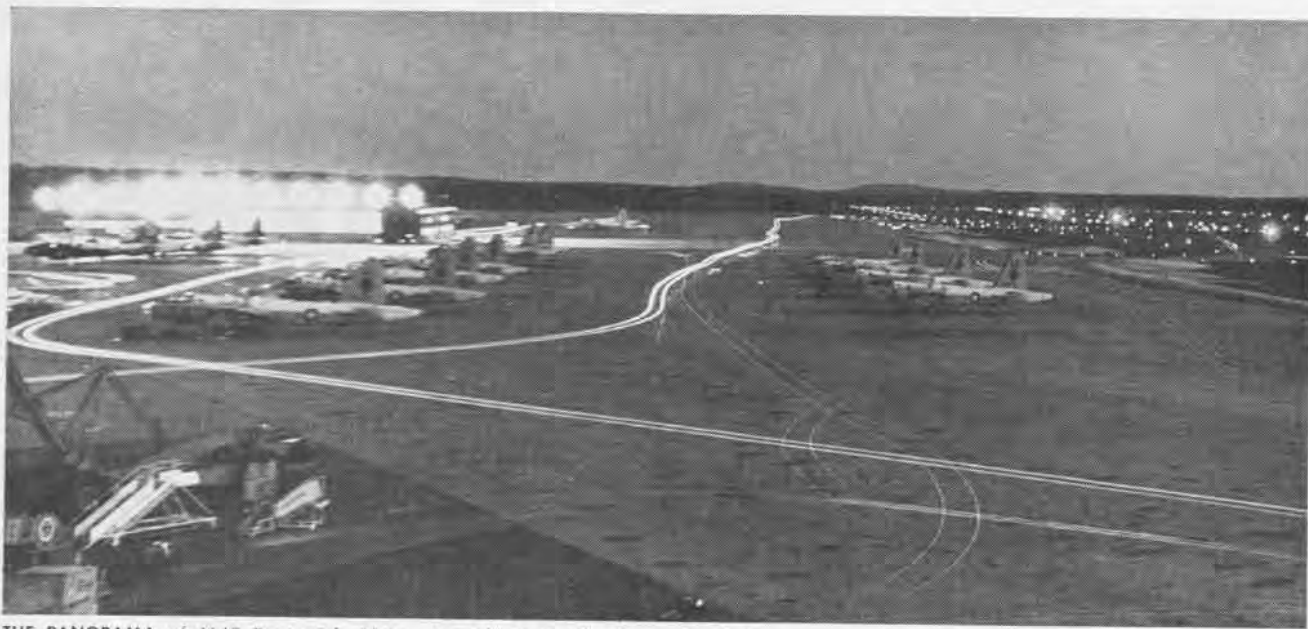
THE PANORAMA of NAS Brunswick, Maine, at night is vividly depicted in this time exposure by Navy Photographer Tom Jones, who slowed his camera speed to capture the trail of lights left by a taxiing aircraft. Photos were taken as the station turned 22 years old.
