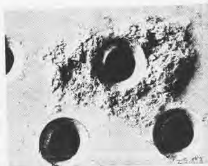
SEVERE CORROSION damage is a condition frequently found adjacent to fastener holes.
