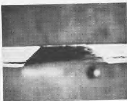
SECTION of an area where fastener was installed: note corrosion parallel to the surface.
