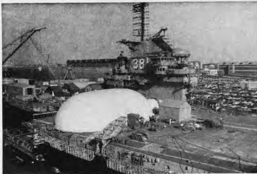
RESEMBLING a gigantic igloo, a vinyl-coated nylon "bubble" set on the flight deck of USS Shangri La enables yard workers to complete jobs in spite of bad weather.
