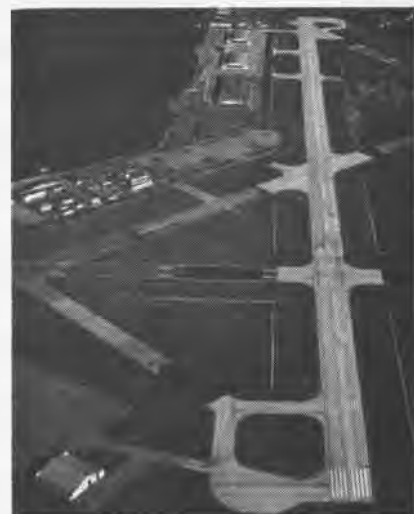
AERIAL OF ELIZABETH CITY RUNWAY
