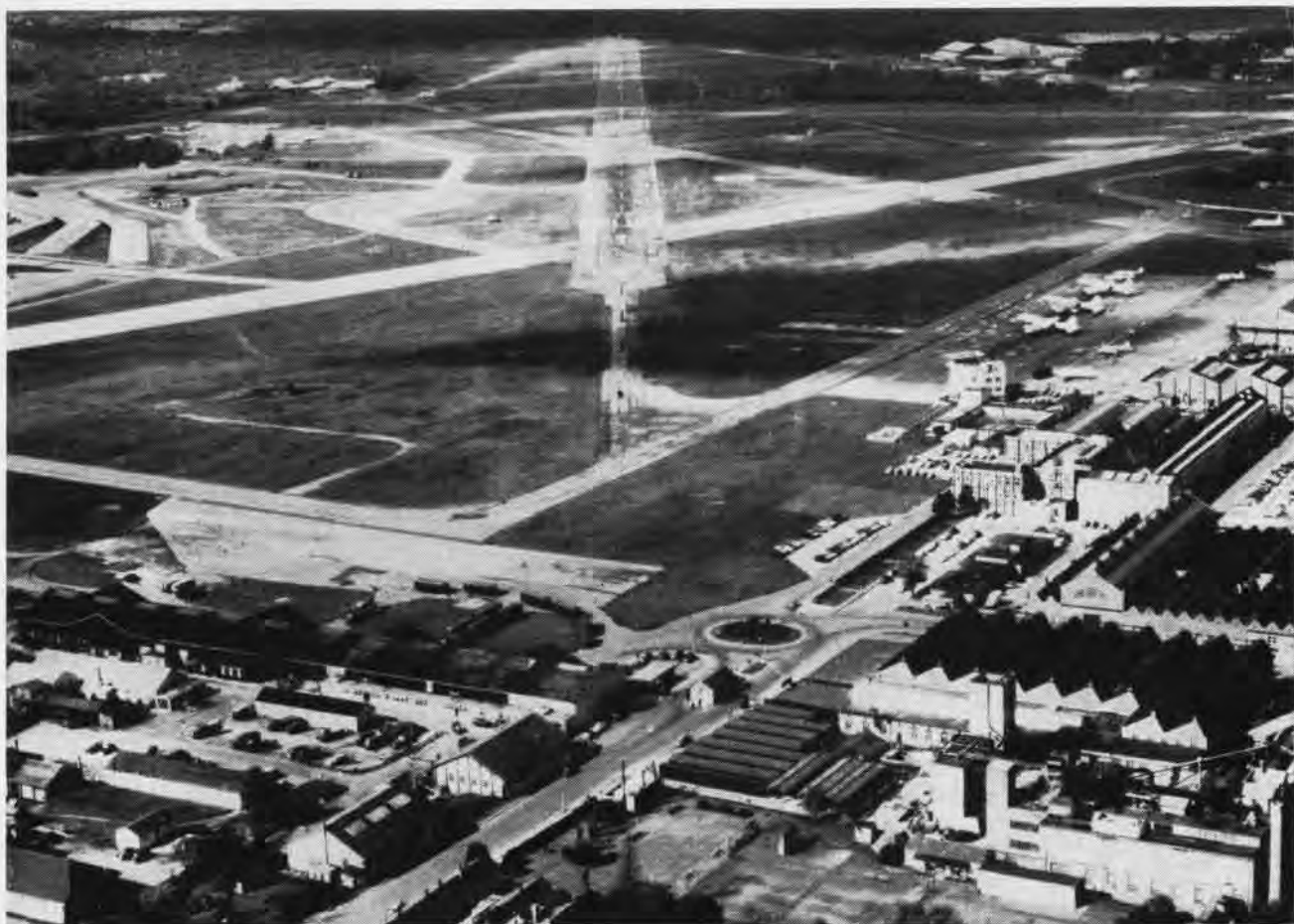
ROYAL AIRCRAFT ESTABLISHMENT, FARNBOROUGH. EMPIRE TEST PILOTS' SCHOOL IS IN BACKGROUND AT LEFT
