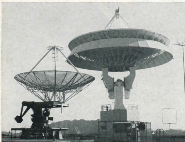
GIANT ANTENNAS atop Laguna Peak are trademarks of the Navy Astronautics Group. They track and relay information to satellites.
