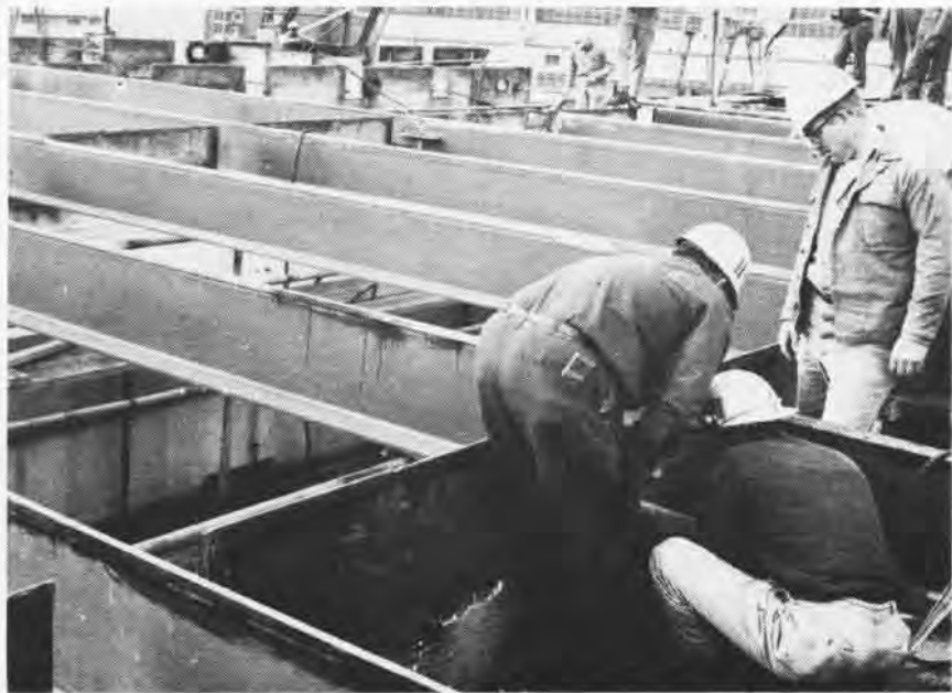
ONE OF FORRESTAL'S damaged five-inch gun mounts is lifted off the ship while she rests in dry dock at the Norfolk Naval Shipyard (above); gun sponsons will be modified for new weapons to be added at a later date. Ship's number four elevator was also removed. In photo below, steel beams are put in place to support new flight deck. Some 800 tons of 1 \frac{3}{4} " steel were ordered to replace portion of flight deck.
