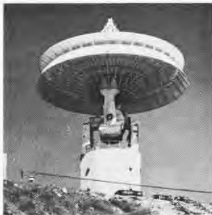
LAGUNA PEAK FACILITY DISH ANTENNA
