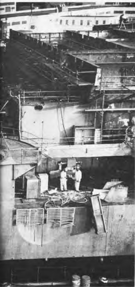
ONE OF FORRESTAL'S damaged five-inch gun mounts is lifted off the ship while she rests in dry dock at the Norfolk Naval Shipyard (above); gun sponsons will be modified for new weapons to be added at a later date. Ship's number four elevator was also removed. In photo below, steel beams are put in place to support new flight deck. Some 800 tons of 1 \frac{3}{4} " steel were ordered to replace portion of flight deck.
