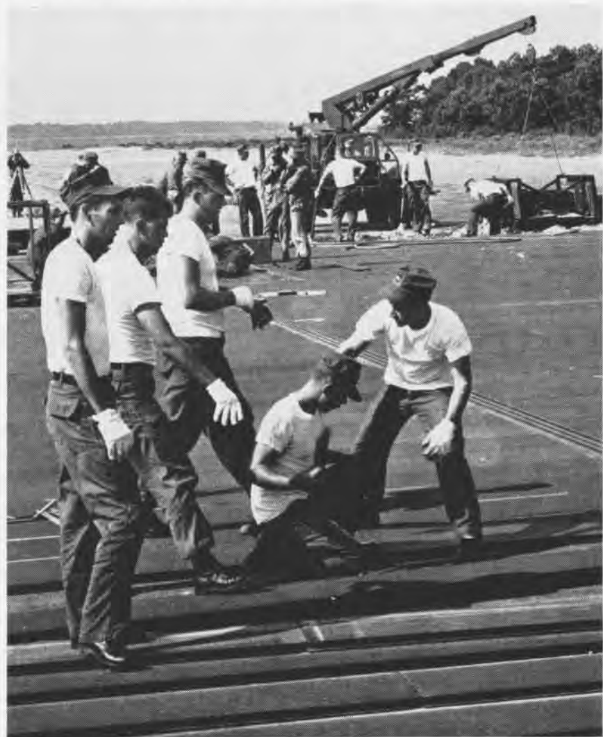
SEABEES LAY SATS MATTING AND CATAPULT TRACK AT THE SAME TIME
