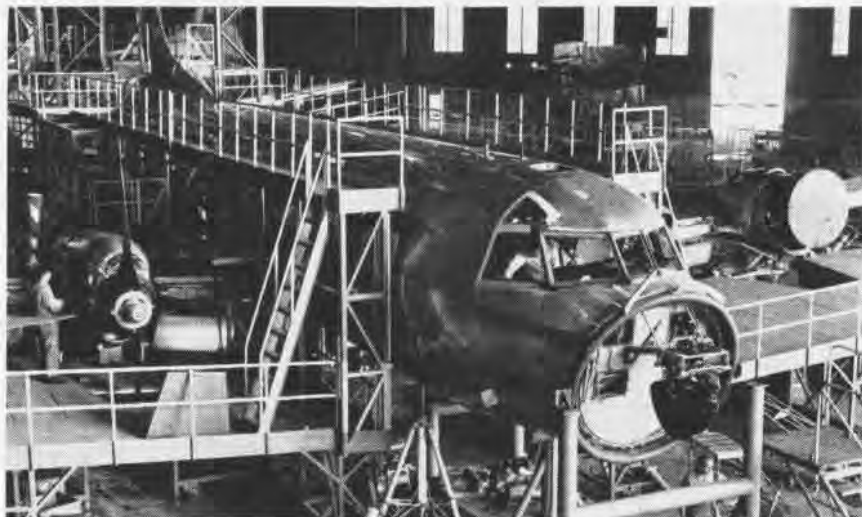
THE P-3 DOCK AS IT LOOKED ON FIRST DAY OF OPERATION AT ALAMEDA
