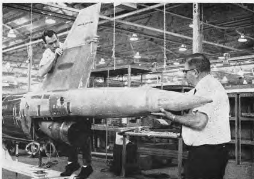
ENGINEERS CHECK PARACHUTE CAN AND TAIL CONE ON FIREBEE II
