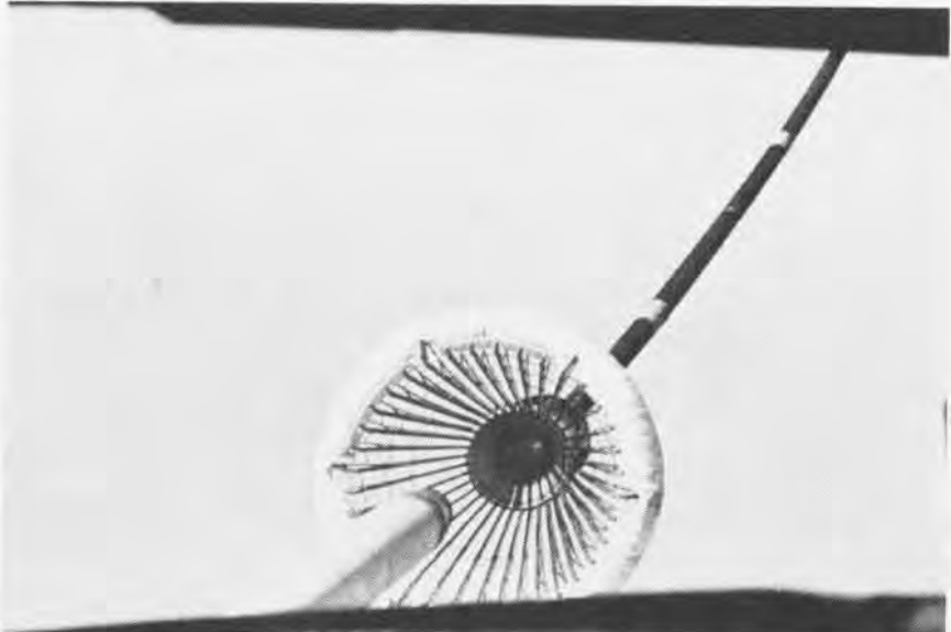
AIRCRAFT INCHES ITS REFUELING NOZZLE INTO THE FUEL LINE BASKET
