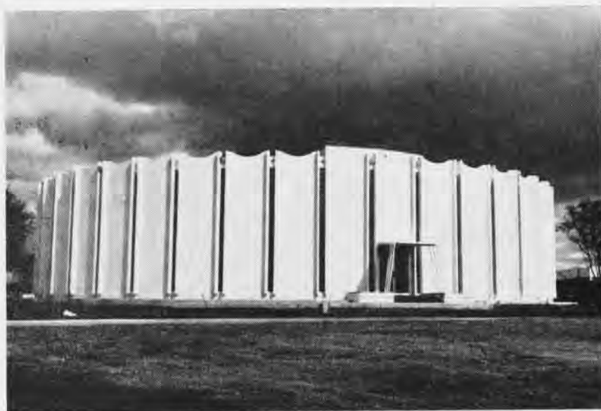
IN JANUARY at Coast Guard Air Station, Barber's Point, Rear Admiral G. D. Synon, Coast Guard Commander in the Pacific, dedicated the nation's first circular military barracks. The revolutionary design grew out of the noise problem at air stations. Flat, rectangular, precast concrete slabs, set at slight angles to each other, deflect sound waves coming from any direction. Construction costs are no more than for a conventional structure. The 150-man barracks has been named the Stone Memorial Barracks in memory of Cdr. Elmer F. Stone, one of the first Coast Guard officers designated a Naval Aviator (No. 38).
