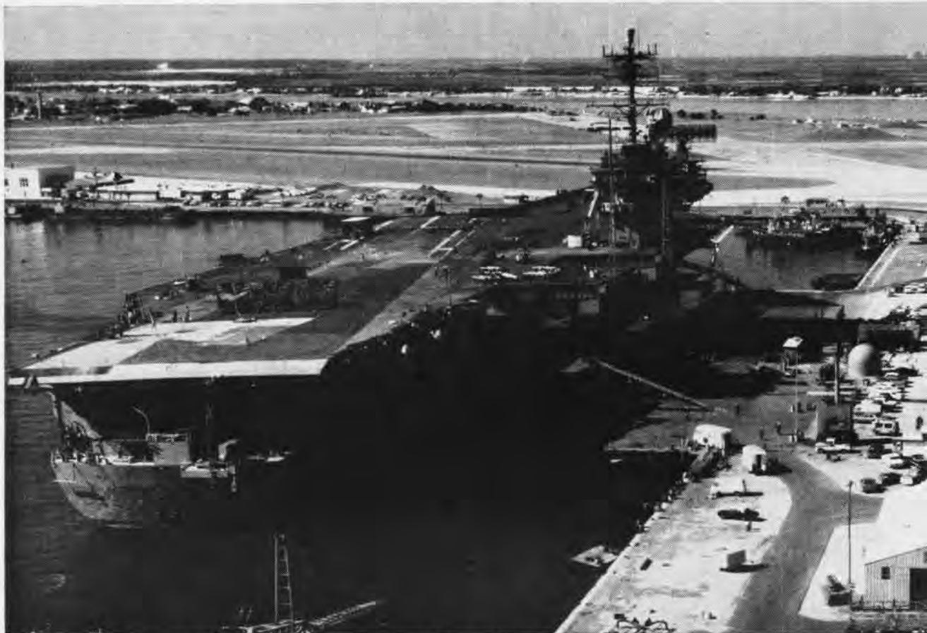
AERIAL VIEW OF USS SARATOGA SHOWS PIERSIDE FACILITIES INSTALLED TO AID SHIP DURING OVERHAUL
