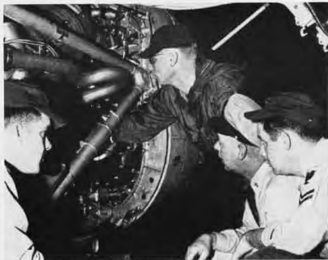
MAINTENANCE MEN TUNE AND TEND ALLISON ENGINES
