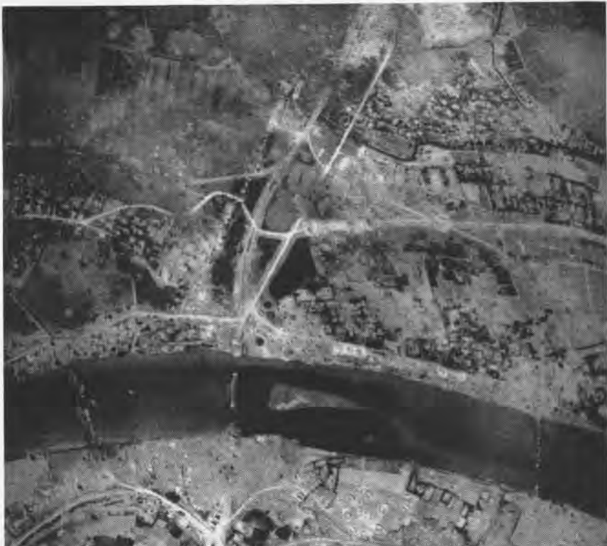
DAMAGE to the Dong Phong Thuong transshipment and storage complex is detailed in post-strike photos. Here, picture shows pontoon and railroad bridges were destroyed.
