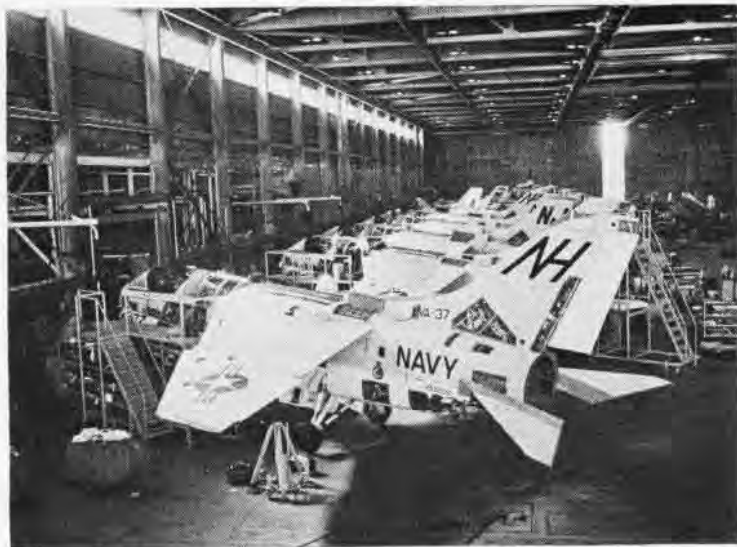
WHILE Cdr. Everett Garrett, NavAirReworkFac Jax production officer (left, in photo above), looks on, Capt. Cyril T. Faulders explains A-7 modernization program to author. Photo at right is of A-7A's on production line. Once they have entered the hangar to undergo required changes, they are not moved until work is done.
