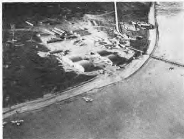
NAS FROMENTINE, FRANCE; CONSTRUCTION BEGAN IN FEBRUARY
