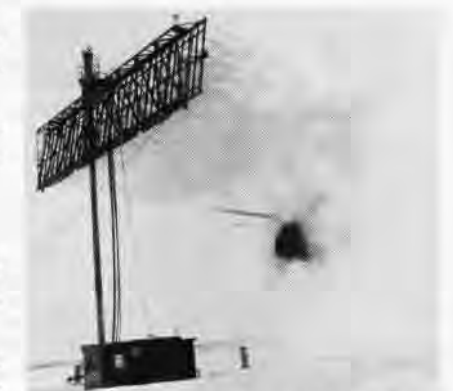
AN SH-3D HOVERS IN ICING SPRAY RIG
