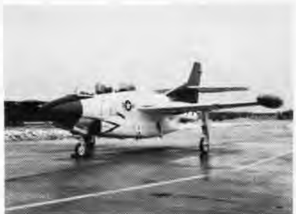
IN FEBRUARY, North American Rockwell Corporation delivered the first T-2C twin jet Buckeye to the Navy. The T-2C looks like the T-2B but has different engines — GE J-85's. It will be used by CNaBaTra.
